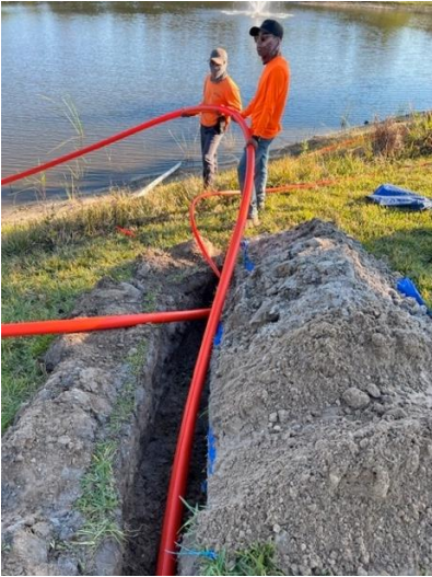
Backbone conduit being pulled
