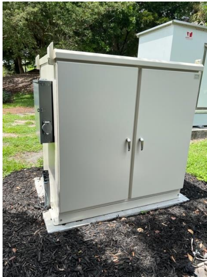
Head-end cabinet to be installed at Aviano and Burgos
