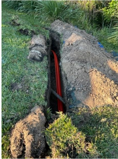
Conduit installed in trench
